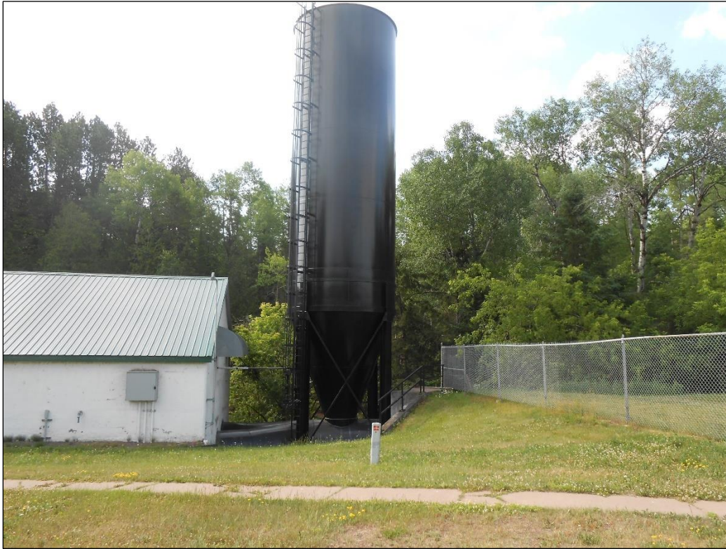
Figure 9.2-3 View of Powerhouse and Surge Tank (looking south)
