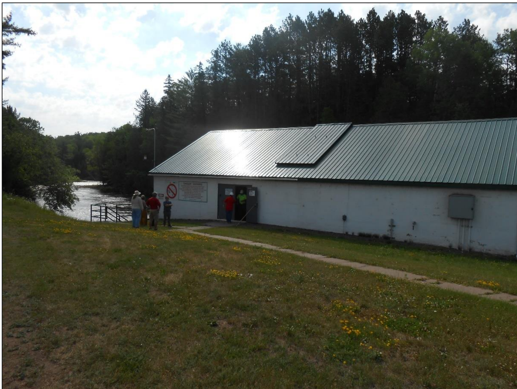
Figure 9.2-4 View of Powerhouse (looking southeast)
