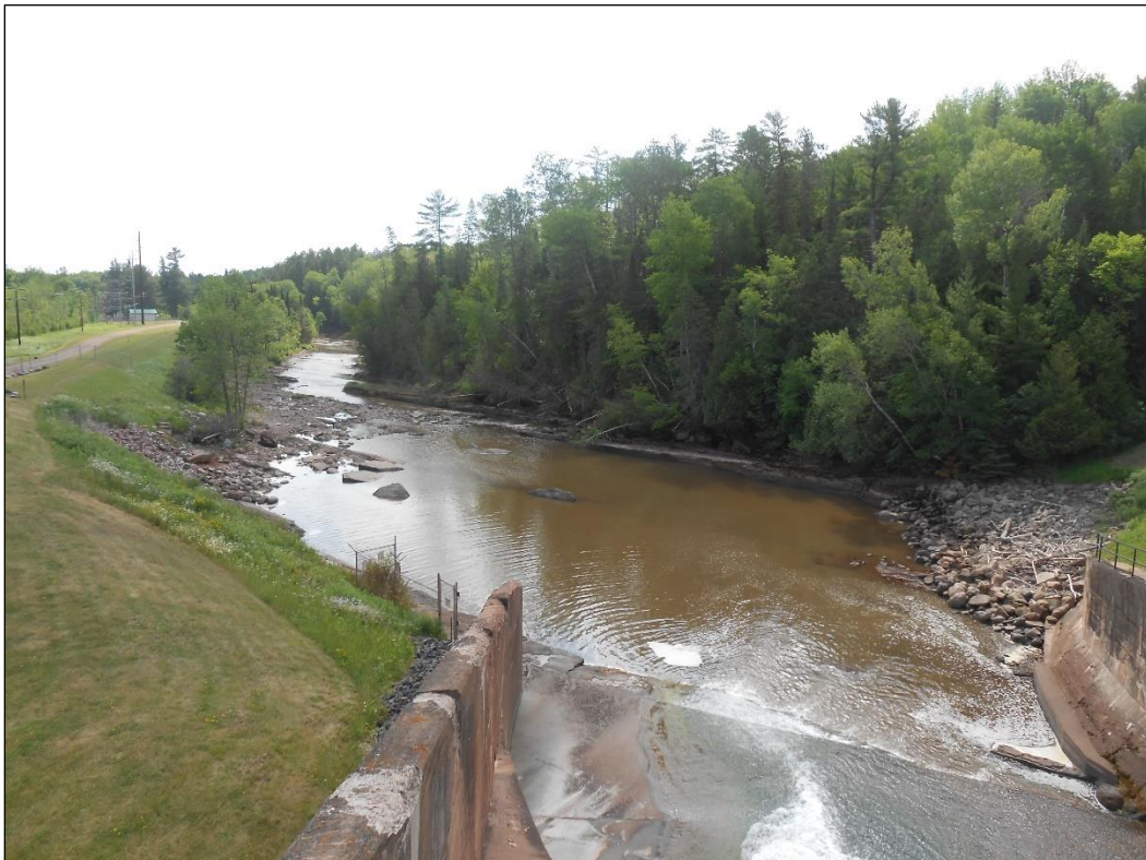
Figure 9.2-2 View downstream of the White River Dam (looking east)
